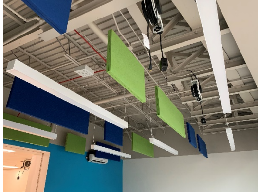
Acoustical Ceiling Baffles In STEM Lab
